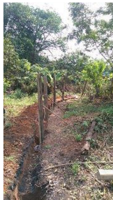
L-R Perimeter fence is walked and marked out. Boundary teak pole positions are measured and marked. Boundary trench is dug and teak poles are cemented into place.
